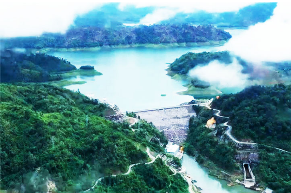
Nam Lik 1-2 administration buildings below:
